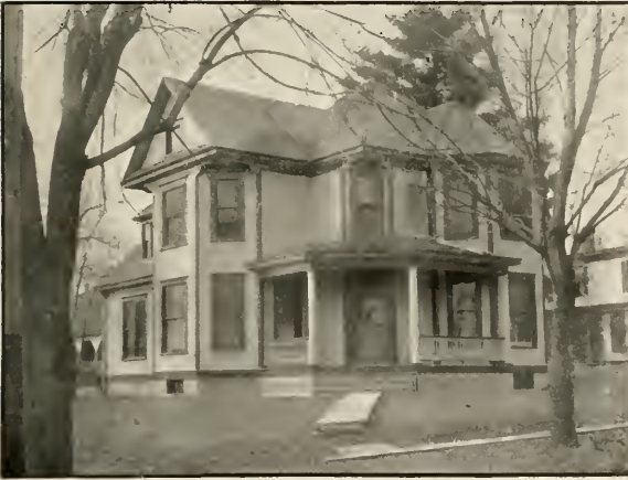
RESIDENCE OF W. A. JOY, East Main Avenue.
