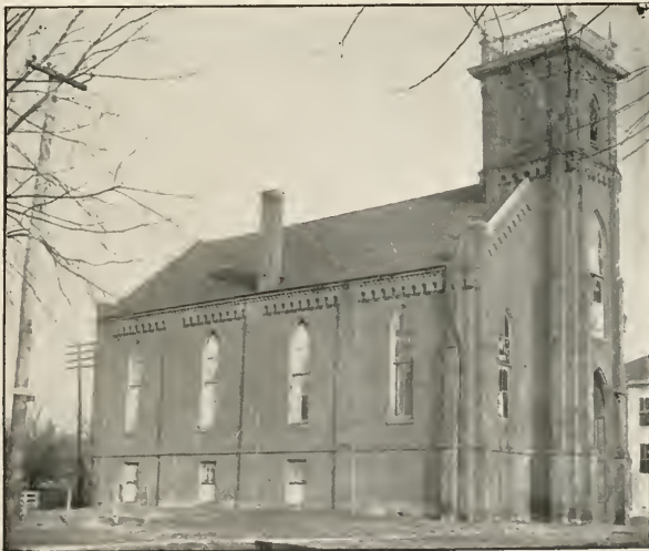
THE M. E. CHURCH, Built in 1877. South Second Street.
