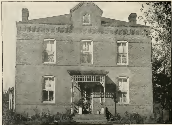
Bond County Jail, built in 1897.
