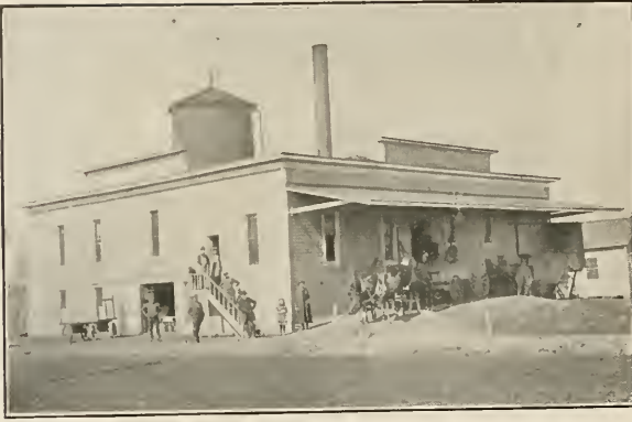
THE PLANT OF THE GREENVILLE MILK CONDENSING COMPANY.
