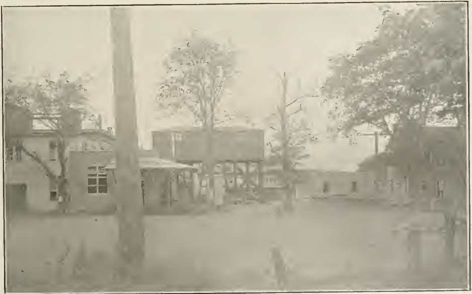
Rear View of a Portion of the Helvetia Milk Condensing Company's Plant.
