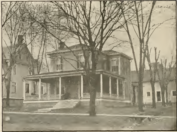
RESIDENCE OF J. F. WATTS, East College Avenue.
